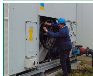
Easily accessible fan drive system at ground level
